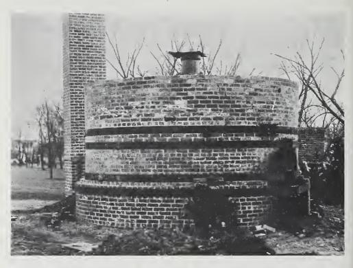
The ceramics kiln was built at Oklahoma A&M College in 1929. All ceramics products manufactured in the ceramics factory were baked in this facility (Oklahoma State Alumnus)
